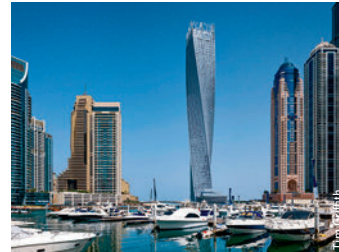
Cayan Tower, Dubai.
